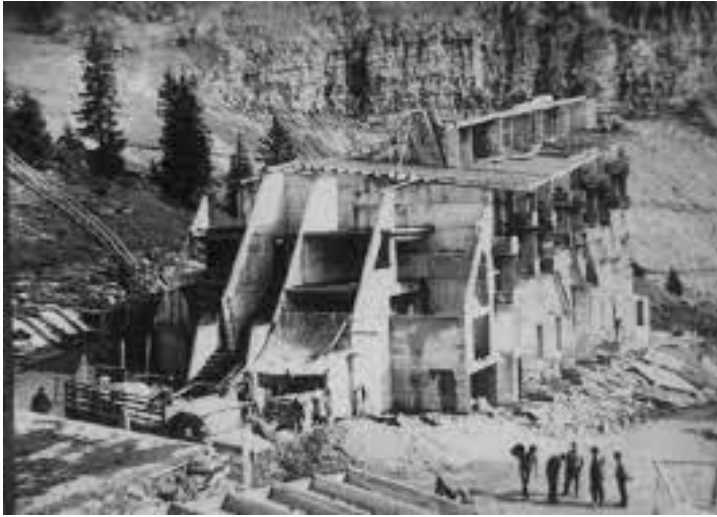
Construction of Avoriaz, 70s
